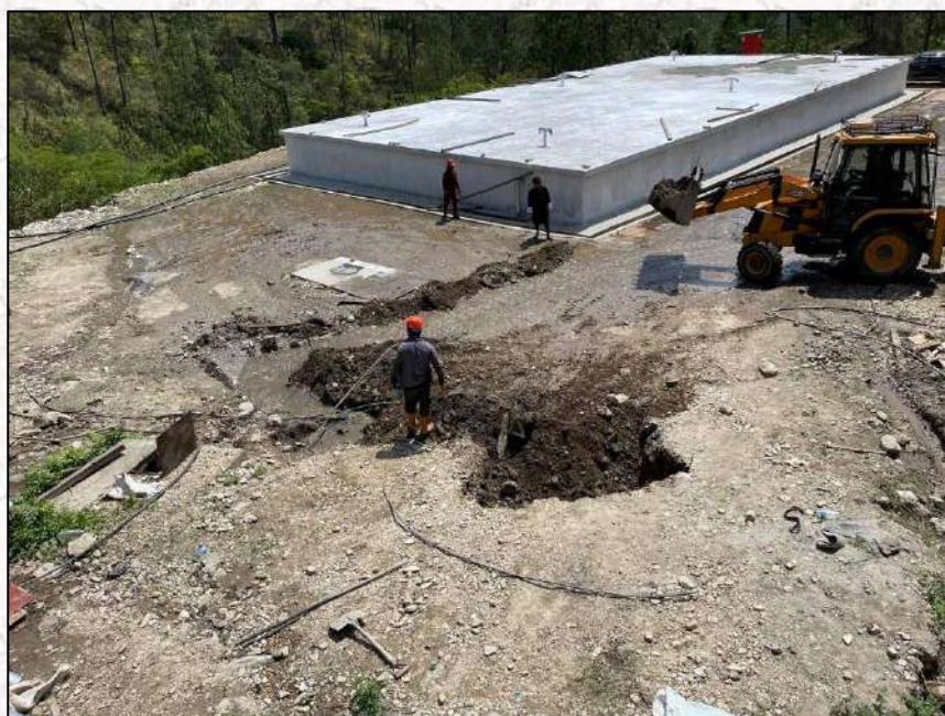
1.03 MLD RCC Reservoir
