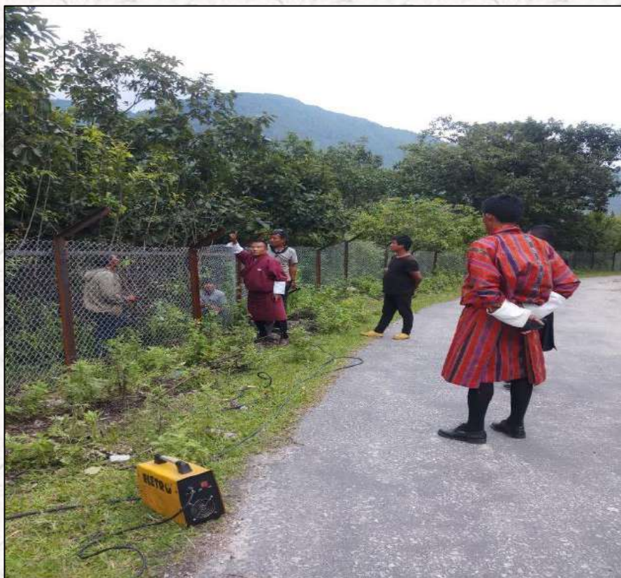
Chain-link Fencing constructed at Nyamed, Ngatshang Gewog
