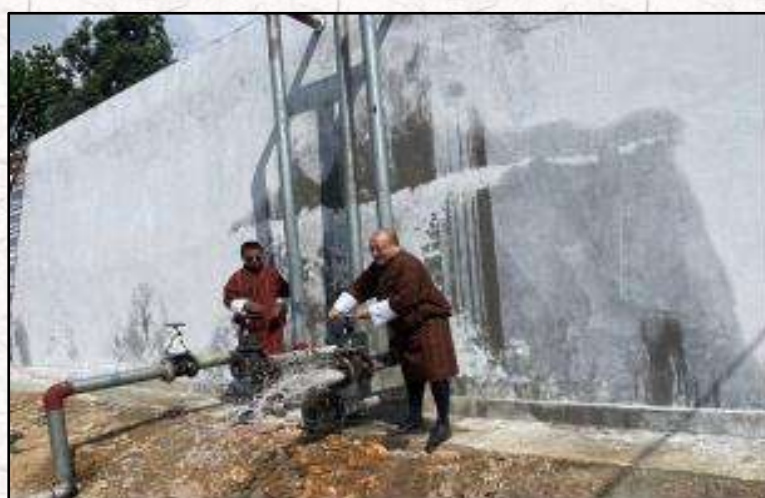
Handing taking of 1.4 MLD reservoir from the contractor
