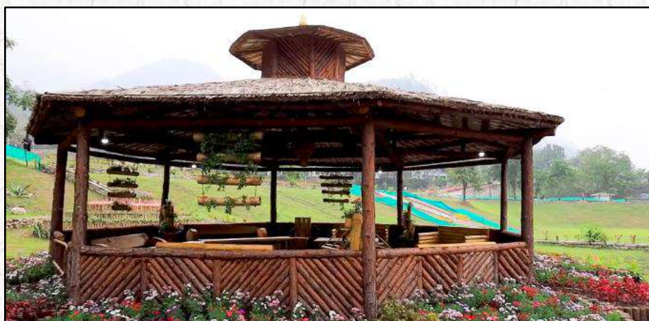
Canopy built from bamboo
