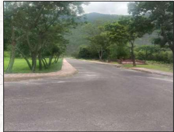
Road & Footpath at Gyelpozhing
