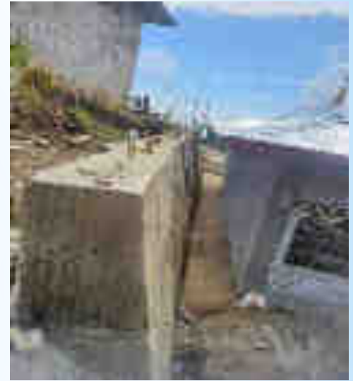
Plum Concrete Wall
